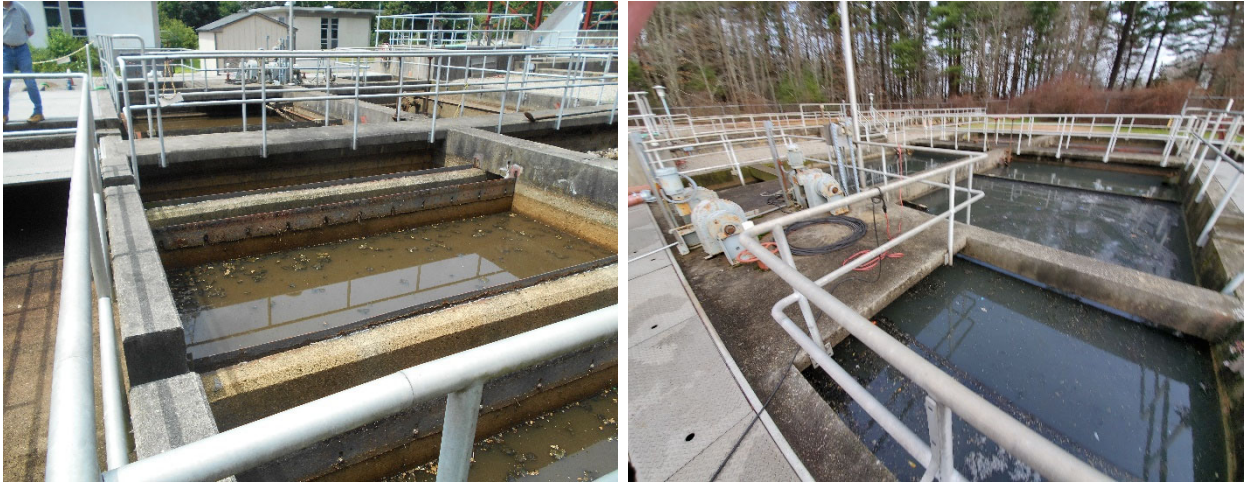
FIGURE 3-12 SMALL PRIMARY SETTLING TANKS
