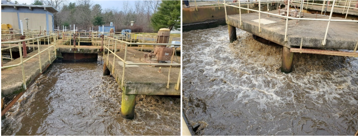
FIGURE 3-14 NITRIFICATION TANKS
