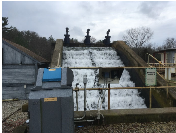
FIGURE 3-22 CASCADE REAERATION STEPS
