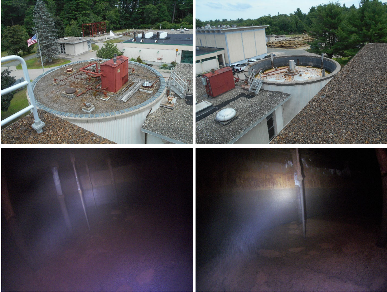
FIGURE 3-28 SMALL ANAEROBIC DIGESTERS
