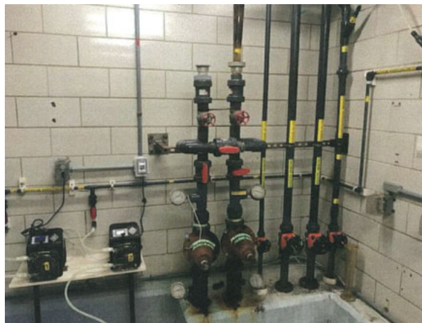
FIGURE 3-24 SODIUM HYPOCHLORITE PUMPS
